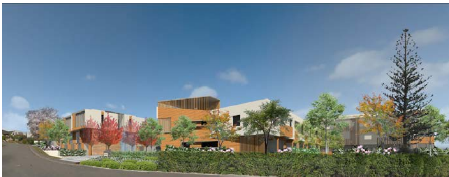
Figure 3 & 4: Rhodes on Cashmere – 31 new Independent Living Units, Communal Facilities and 40 Care Beds
