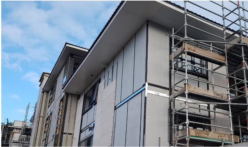
Aria Bay Apartments, Auckland
