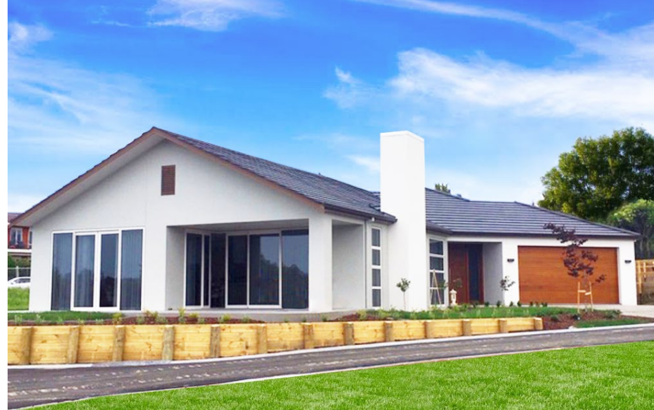
BETHLEHEM COUNTRY CLUB, TAURANGA 2 Villas completed; 1 sale settled 1H20, 1 sale settled 2H20
