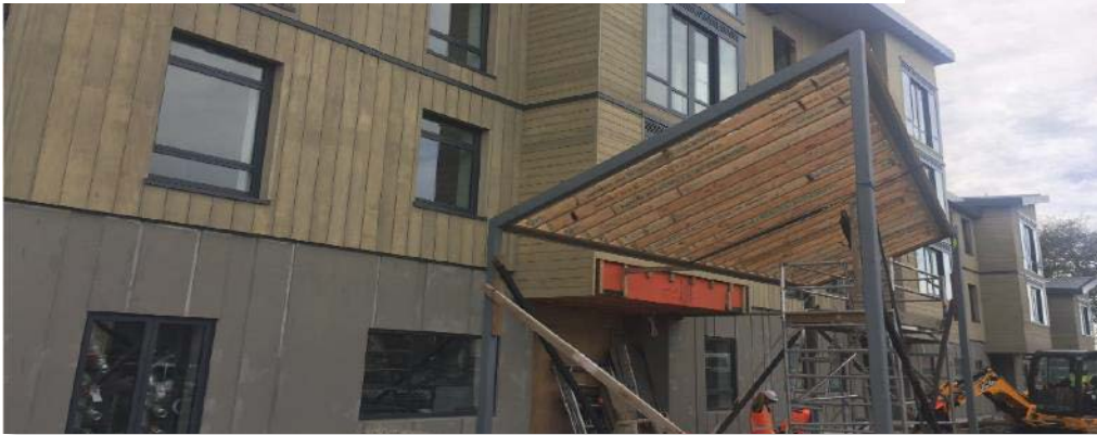
Park Lane Care Apartments - Stage One, Christchurch
