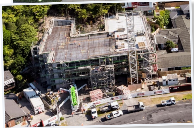
Developments at Aria Bay. Top and centre: Artist's impressions of apartment views and main entrance. Bottom: Construction progress.
