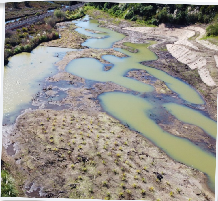
Top: Aria Bay's new care centre exterior is nearing completion. Centre: 29 apartments and 55 care suites are progressing well at Copper Crest. Bottom: Arvida recently completed remediation of the wetland area at Bethlehem Shores.
