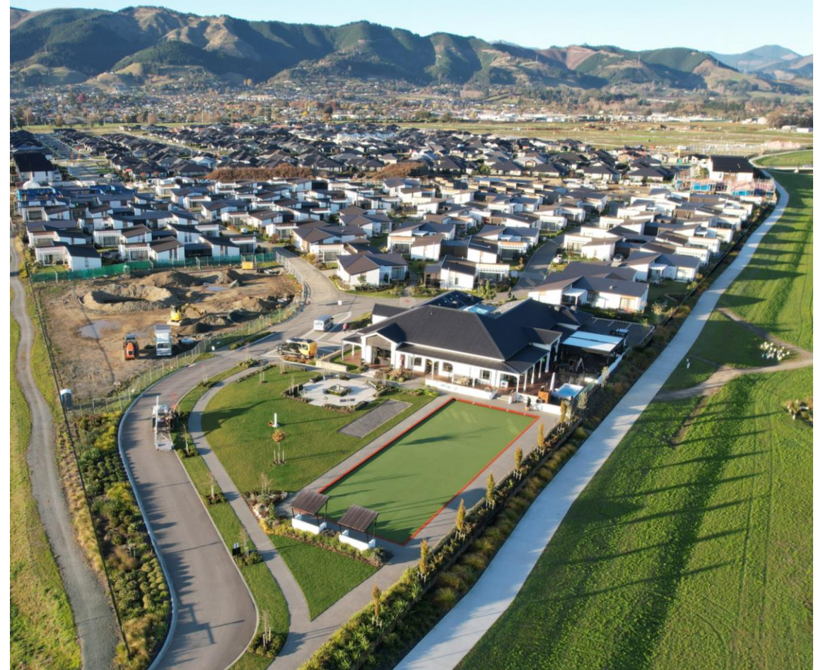
Waimea Plains, Richmond | 120 villas have now been delivered since receiving consents in 2019. Villa construction continues, with a further 66 planned over the next 3-4 years. Pre-construction planning is currently underway on the care centre.
